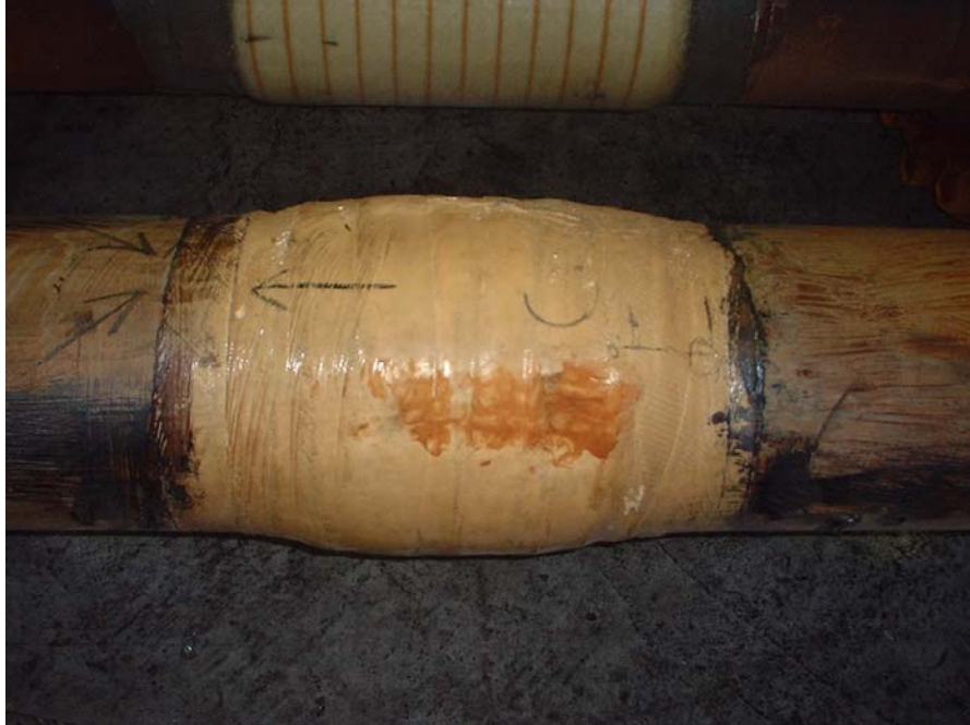
Figure 12 Photograph of Pipe Repair (IMG)
