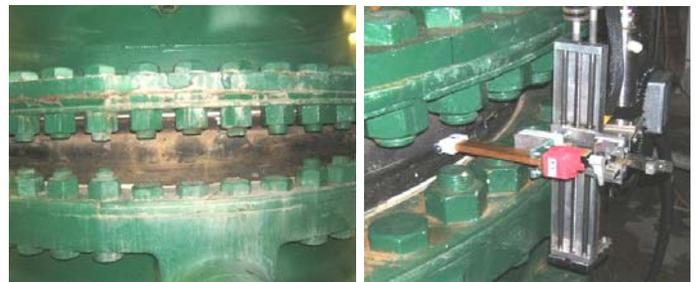
**FIGURE 5: EXPANSION JOINT WITH SCANNING EQUIPMENT**
